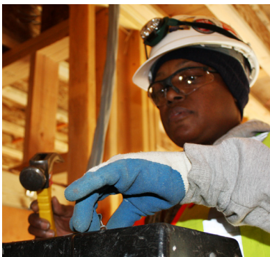
Electrical apprentice Angela Rivers earns while she learns.
