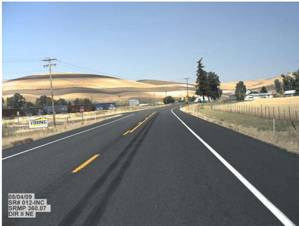
Figure 8-5: Segment photo at ARM= 356.77, US 12
