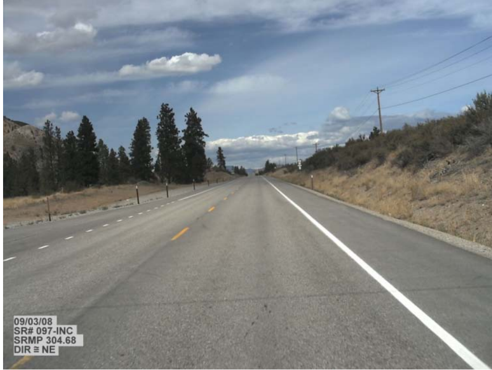
Figure 8-4: Segment photo at ARM= 289.57, US 97
