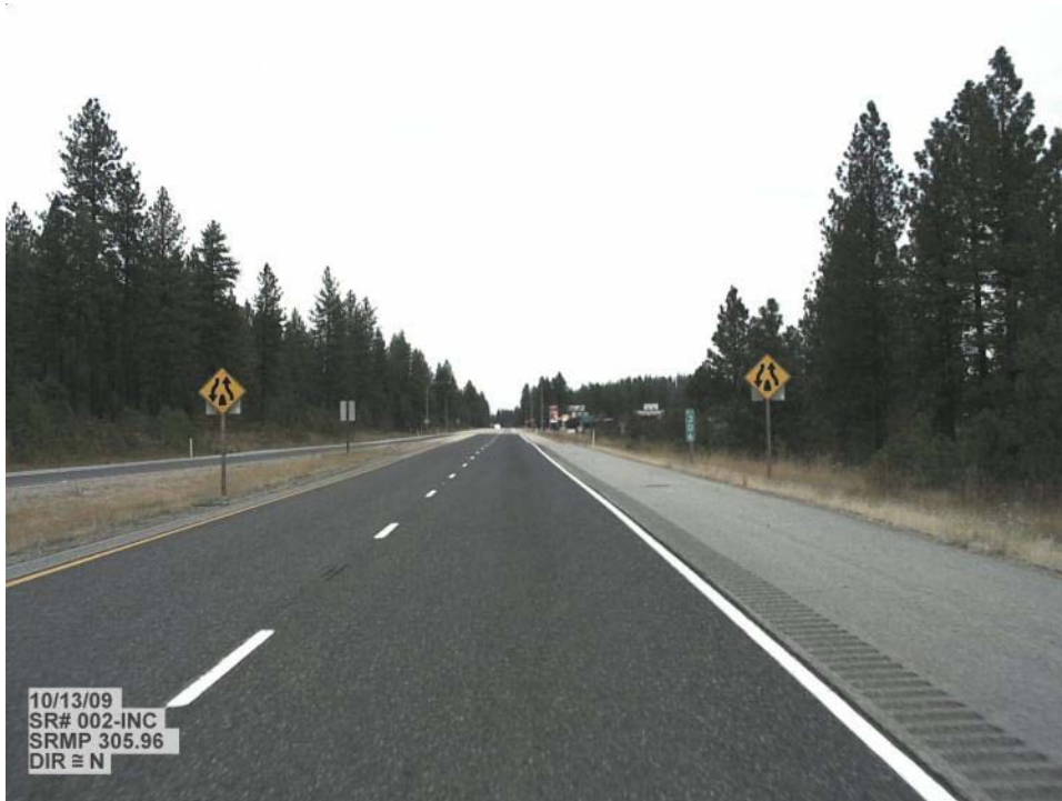
Figure 8-3: Segment photo at ARM= 297.88, US 2
