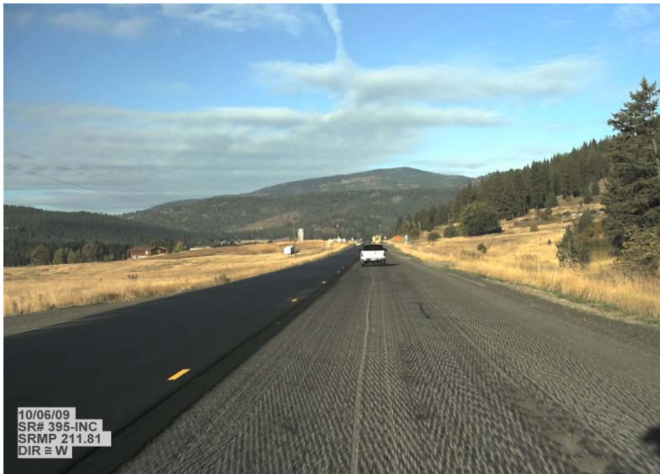
Figure 8-7: Segment photo at ARM= 216.6, US 395
