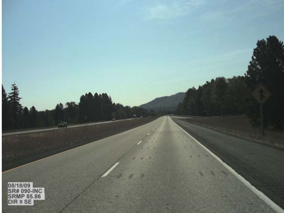
Figure 8-6: Segment photo at ARM= 84.15, I-90
